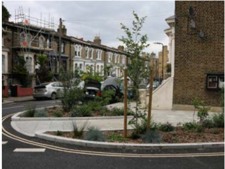
Recent SuDS replacing car parking spaces on Wilton Way have improved the overall street environment and safety.
