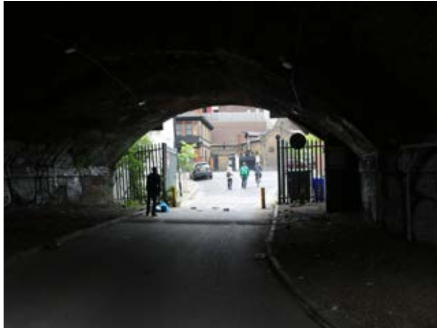
Some connections under the railways are uninviting and would benefit from improved public realm design and lighting to curb anti-social behaviour.
