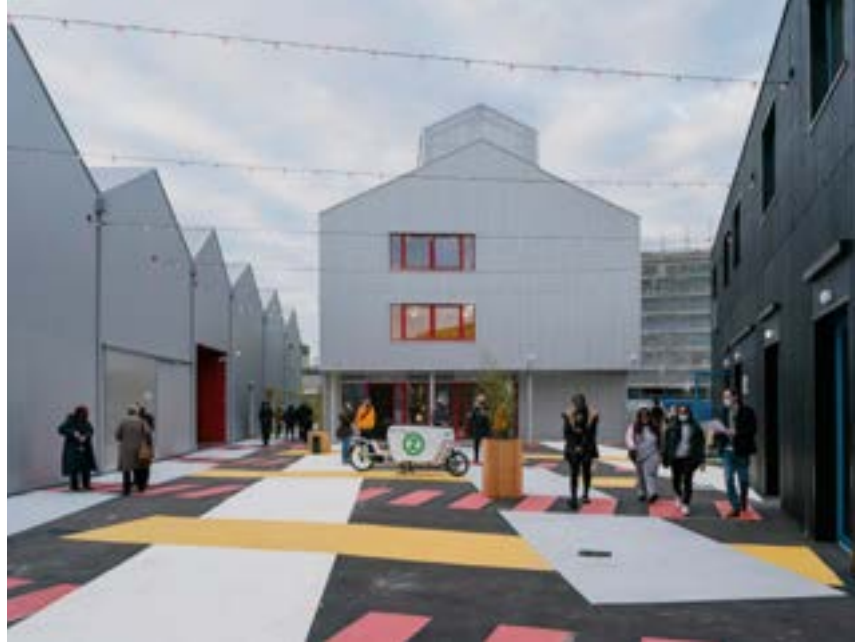
Hackney Bridge in Hackney Wick, designed by Turner Works for Make Shift, is a temporary, meanwhile use project that provides with workspace, incubator space, event space, food halls, and public space. The buildings have been designed to be easily dismantled. Photo by Tim Crocker.
